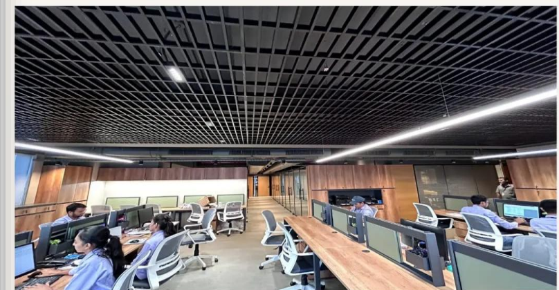
SUCCESSFULLY DELIVERED THE PROJECT ON TIME OF VRF - HVAC
