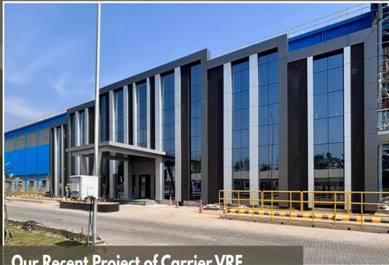
Our Recent Project of Carrier VRF @ TATA Steel Downstream Products LTD
