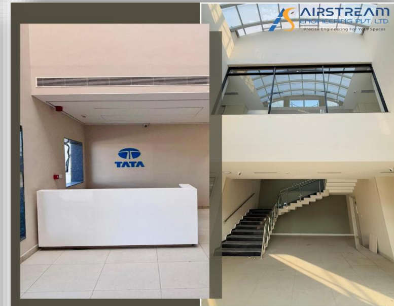
Our Recent Project of Carrier VRF @ TATA Steel Downstream Products LTD
